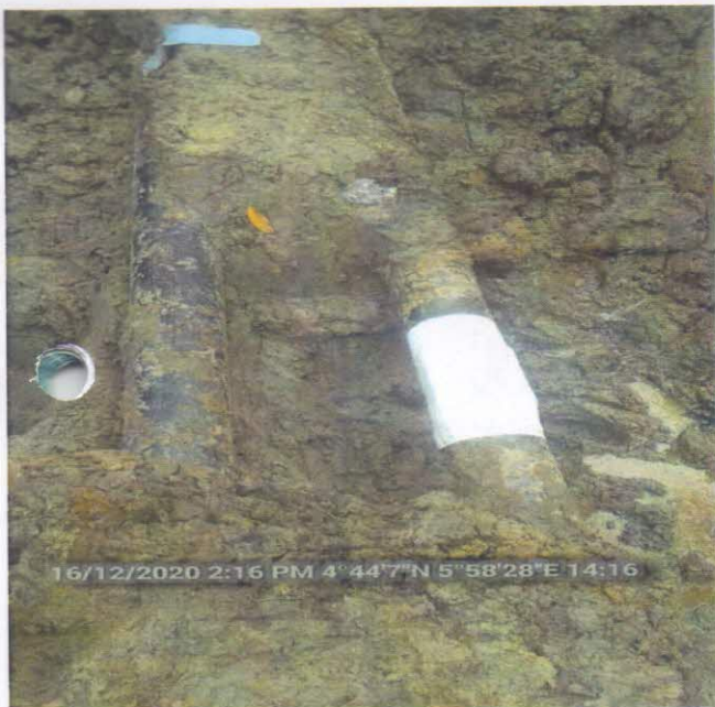
Fig C: Incident facility after repair
